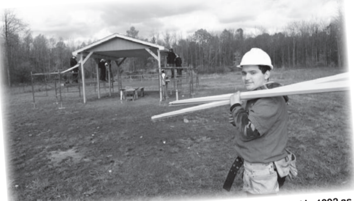
The Construction & Building Maintenance program was added in 1992 as "Buildings & Grounds." Here, Carlos Matos gains valuable field experience at a jobsite in Pierpont in 2018. PHOTO BY CARL E. FEATHER
